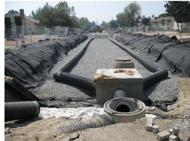
Mixing and Immediate Discharge
